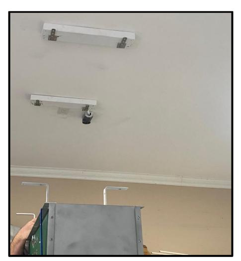
The enclosure side panels have four (4) hanging brackets attached. Two (2) persons using ladders lift the enclosure and slide the enclosures' hanging brackets into the ceiling slide-in brackets. The enclosure's total weight is about 72 lbs. (33.6 Kg). The power cords extending from the rear of the enclosure are plugged into the ceiling outlets.
